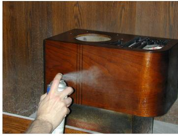
Figure 17: Spraying the clear coat.
